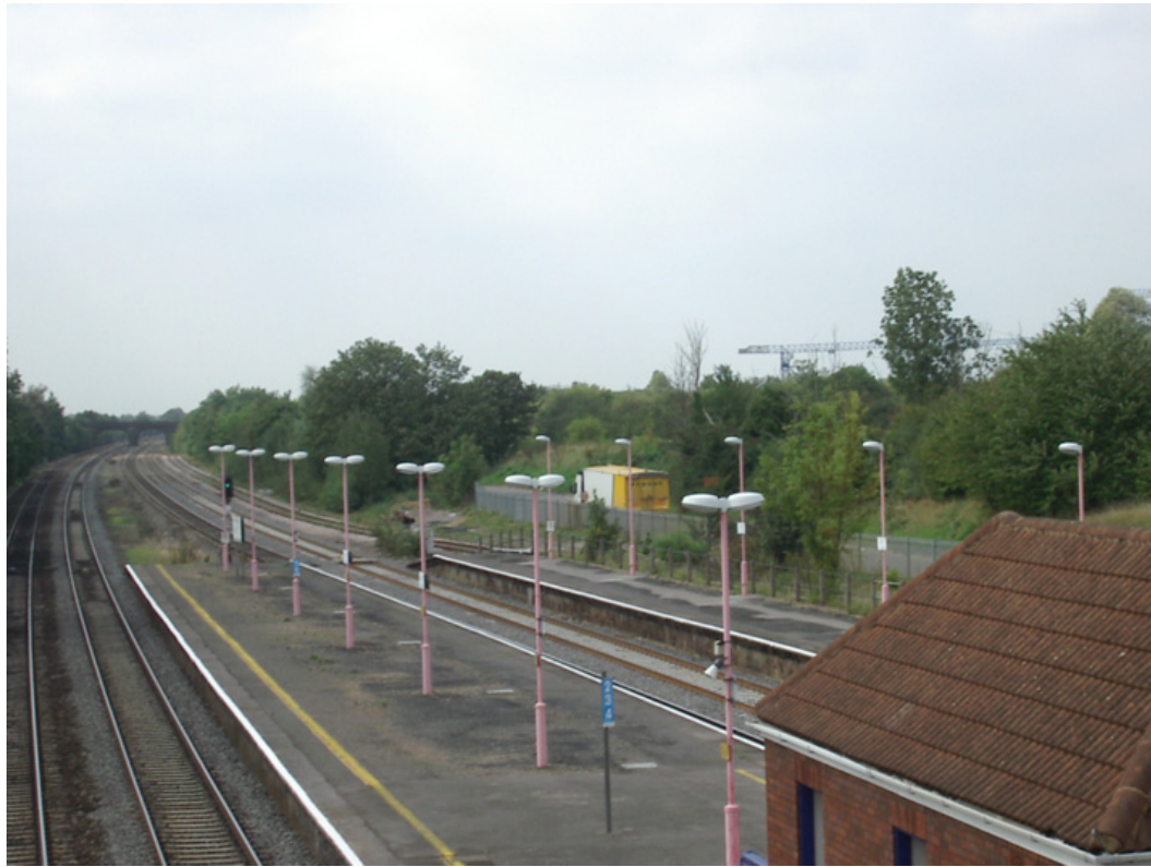
Figure 13.2: Location of Iver Station worksite – north of platform 4
