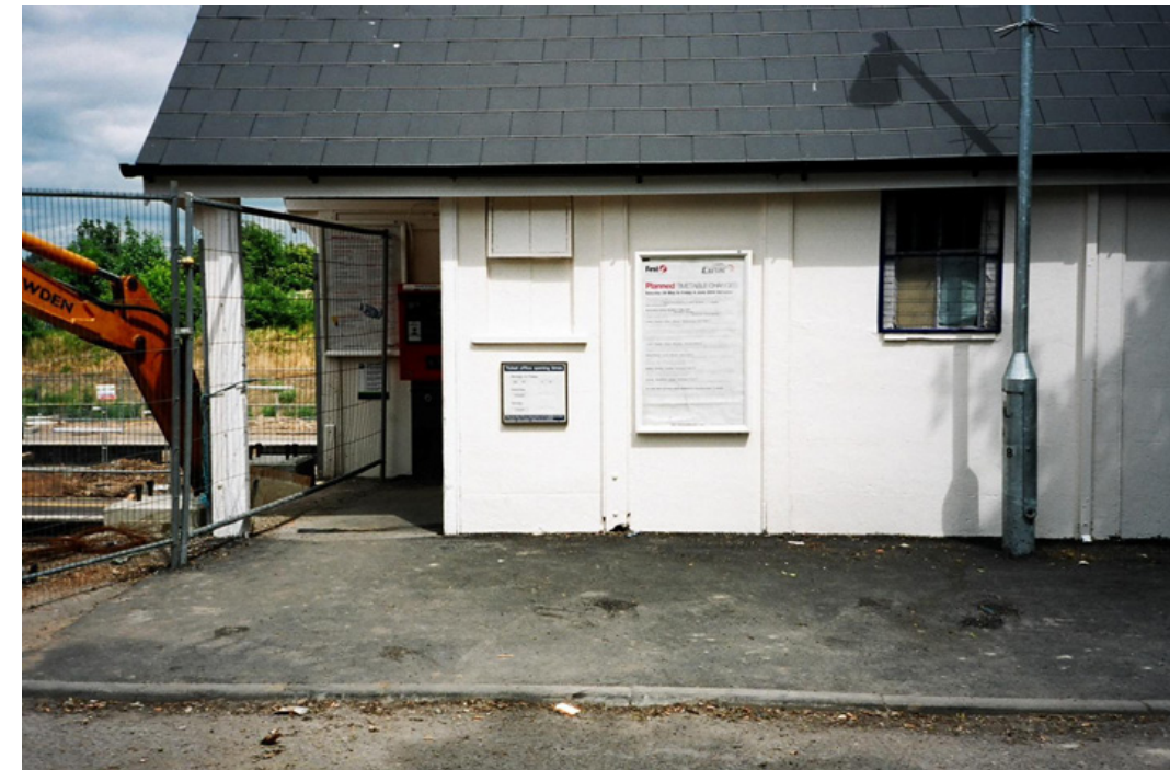
Figure 13.1: Iver station entrance
