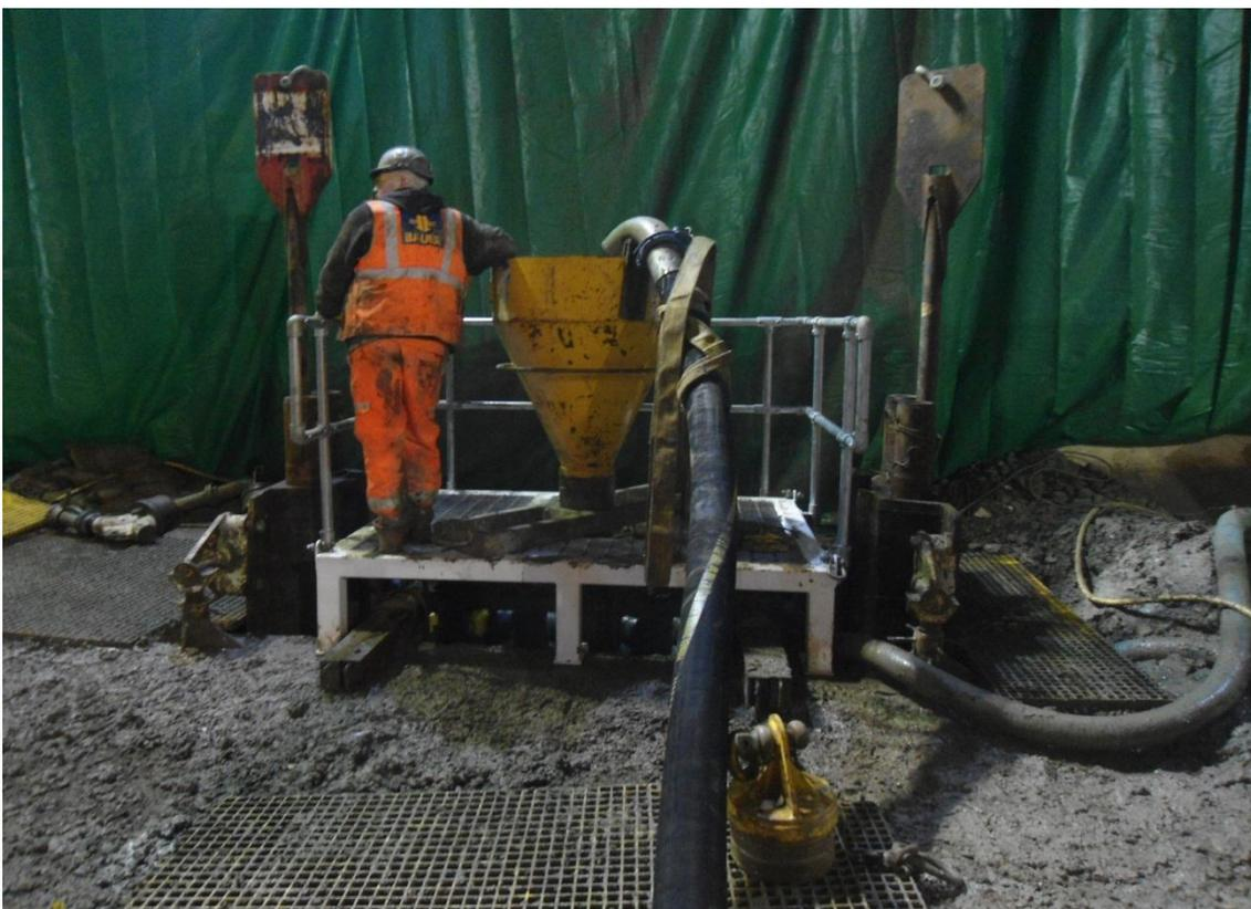
BAUER concreting platform during installation of the diaphragm wall panel from the low level working platform at Whitechapel, Durward Street Shaft.
