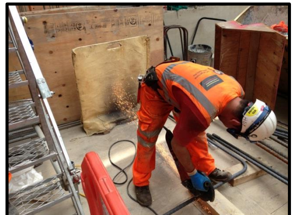
Sparks landing on portable screen
