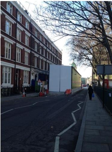
Any noise from concrete deliveries and pumping operations will be mitigated at source by housing these activities within an acoustic enclosure adjacent to Charterhouse Square (see photo).
