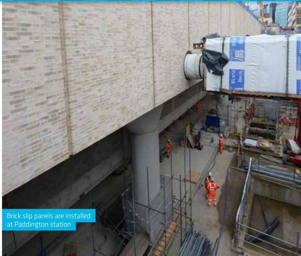
Brick slip panels are installed at Paddington station
