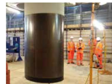
Bronze cladding is fitted to the station's columns
