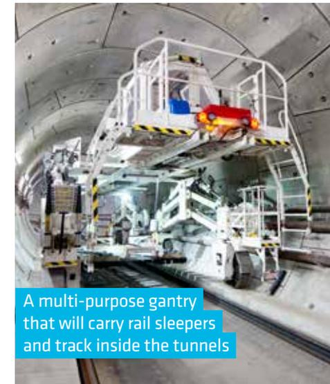
A multi-purpose gantry that will carry rail sleepers and track inside the tunnels
